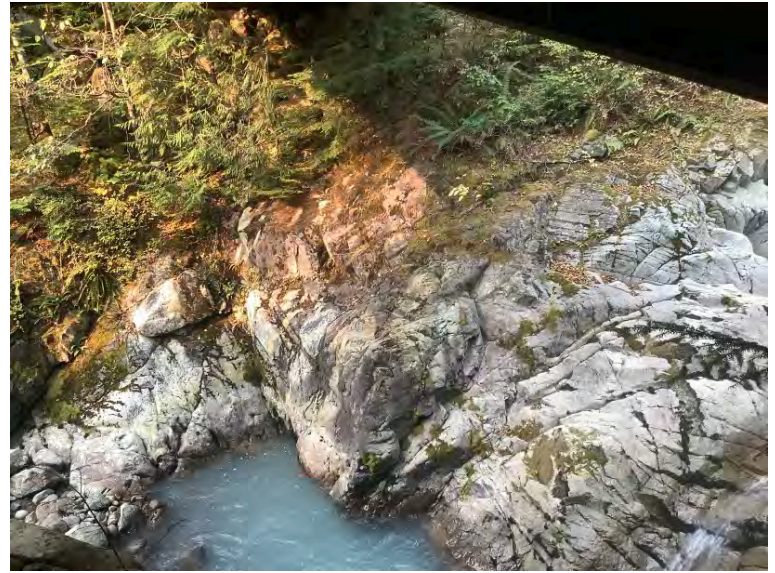
Right Bank Abutment when facing downstream
