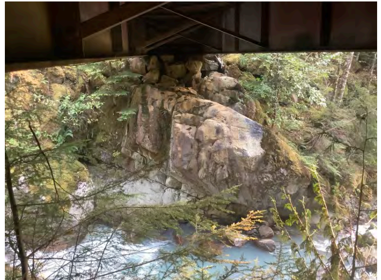
Left Bank Abutment when facing downstream
